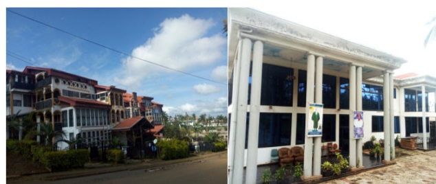
Figure 4 and 5: Showing a Mansion constructed at Bamendankwe and Late Lawyer Sama's House at Virgin land, Foncha Street
